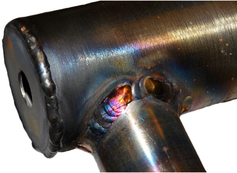
Figure 10 Typical recumbent frame fatigue failure along the chainstay weld.
