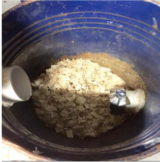
Figure 6: Second Filter, “dry filter”. Once filled with wood chips, the gas will be pulled through the wood chips where they will act as a filter.
