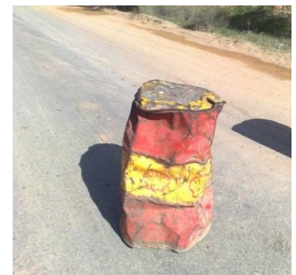
Picture (2) Use of metal drums non good
