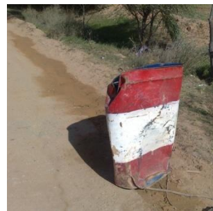
Picture (2) Use of metal drums non good
