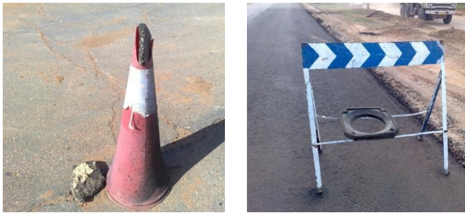
Picture (3) Barriers do not comply with the technical specifications
