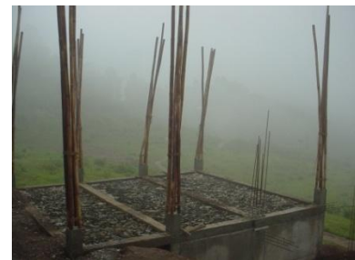
C) CONCRETE GRADE-BEAM FOUNDATION WITH RUBBLE INFILL.
