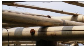
(D) SEVERE SPLITTING INITIATED BY PRESENCE OF BOLTED CONNECTION
