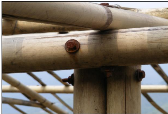
(E) INITIATION OF SPLITTING AT BOLTED CONNECTION
