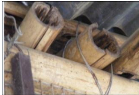
(C) SEVERE SPLITTING AT SAWN ENDS OF ROOF RAFTERS
