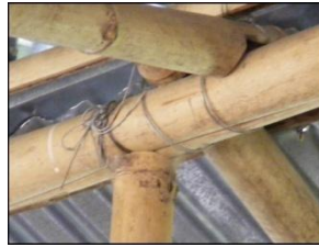
(B) BEAM SPLITTING NEAR SAWN END AT DOWELLED AND LASHED JOINT
