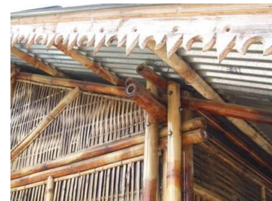
D) BOLTED CONNECTIONS USED TO CONNECT PRIMARY FRAMING.
