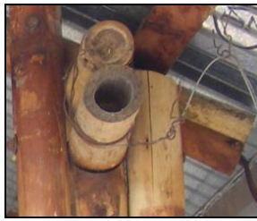
(A) COLUMN SPLITTING NEAR SAWN END
