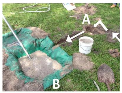
*Figure 4*. Trench pit system, consisting of (A) the settling pit, (B) the mud pit, and connecting trenches dug perpendicular to each other.
