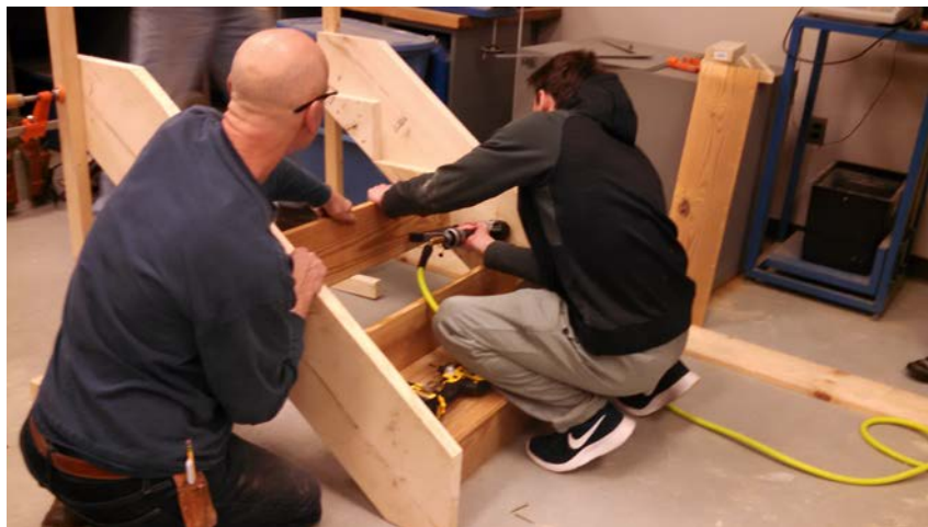
Figure 1 Student working with master carpenter building stairs in final lab.
